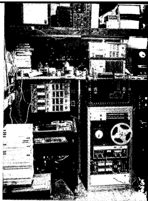
Fig. 2. Radio booth, backstage at first balcony level of Symphony Hall, houses five tape recorders, monitor loudspeakers, and other gear including oscilloscope for checking phase and stereo/mono content.
